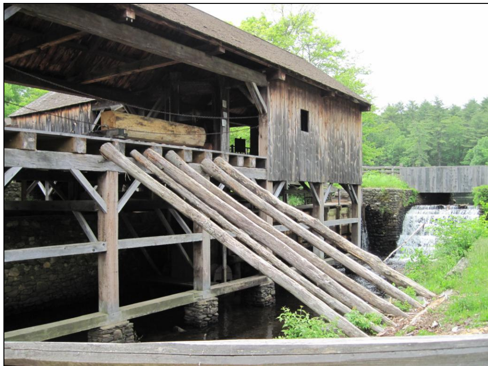
Figure 14: This water-powered sawmill uses a box sluice rather than a waterwheel, but the construction and the up-and-down saw are typical of the 1830s. (D. Heyduk photo, Sturbridge Village)
