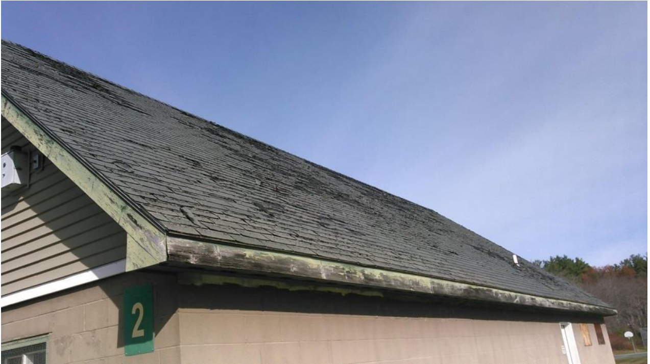
Lower Prescott Park Restroom Building Roof Replacement and Other Repairs Required
