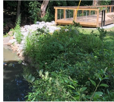
Erosion Control: Restoration Planting / Live Stakes
