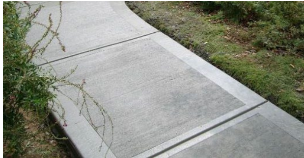
Cast-in-Place Concrete Pavement
