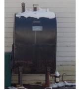
underground. All above ground storage tanks according to code, whether outside or inside, should be pitched ¼ inch per foot toward its opening so as to minimize the potential for corrosion. The best remedy, for those with a cellar, is to move the outside tank inside and have the appropriate safety devices installed. Lacking a cellar the choices get more expensive. An aboveground double-walled tank with a weatherproof cover is available for
